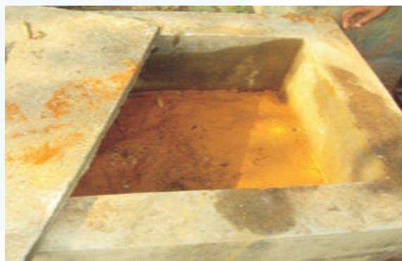
Arsenic Contaminated Sludge Collection
