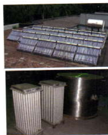
Figure 3: Solar Water Heating System and Sorption Heat Exchangers at CMERI
