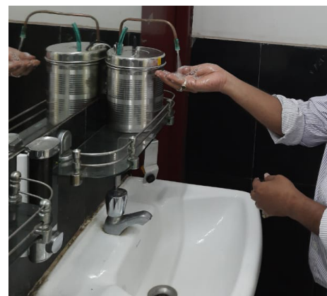
Installed at CSIR-CMERI Guest House
