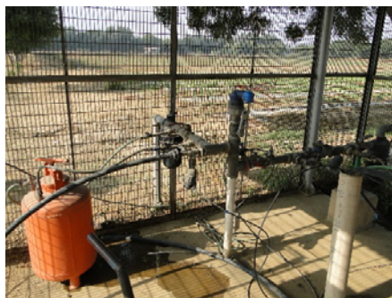
Fig 1: Irrigation Head Control Unit for Pressurized Drip Fertigation System
