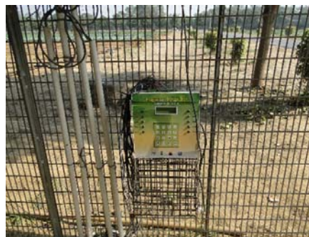
Fig 1: Irrigation Head Control Unit for Pressurized Drip Fertigation System
